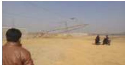
HT Tower falling down after the earthquake
