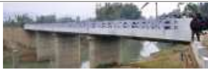
Keirao Litan Makhong Bridge inaugurated by Works Minister today
