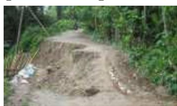
The condition of the roads here is no better. In some parts, the roads have been damaged heavily by rainfall and resultant landslide and using them can be quite risky. In some parts, deep craters have formed in the roads.
