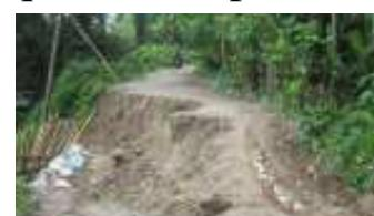
The condition of the roads here is no better. In some parts, the roads have been damaged heavily by rainfall and resultant landslide and using them can be quite risky. In some parts, deep craters have formed in the roads.
